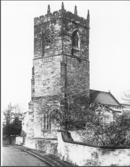
Aston church tower with a missing pinnacle
